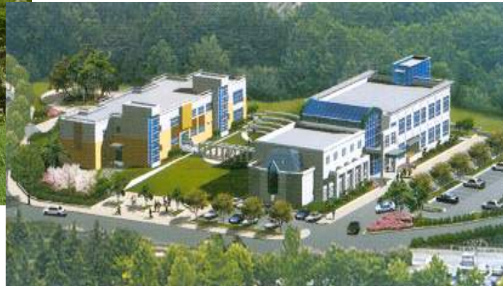
NTC's INTEC Building
