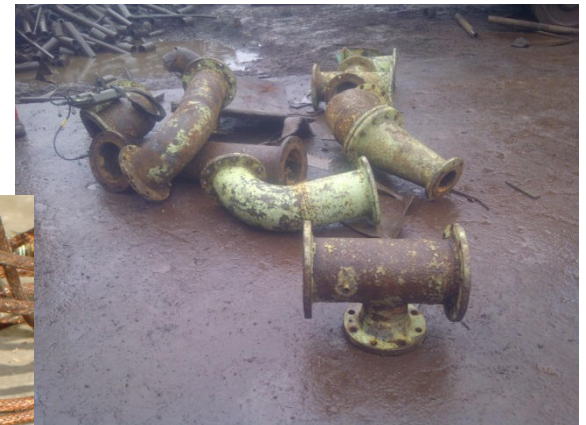
Pipeline with mineral residues containing Ra-228sec
