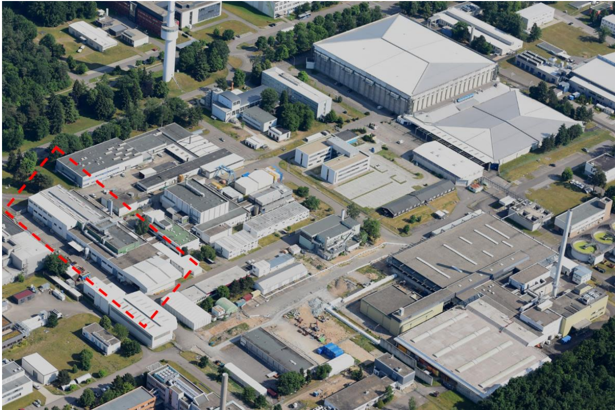
Figure 5. Aerial view of the plant as a start of the slide show substituting the site inspection.
