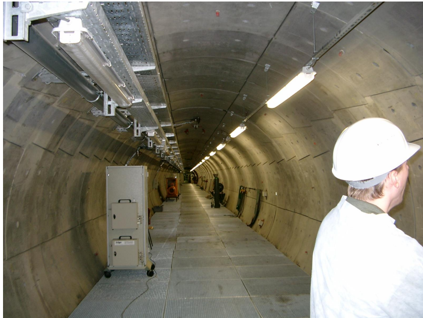
Fig.2: The underground laboratory HADES in SCK•CEN, Mol
