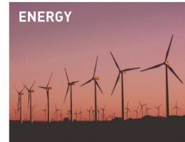
ENERGY EDP | IBERDROLA | ENGIE
